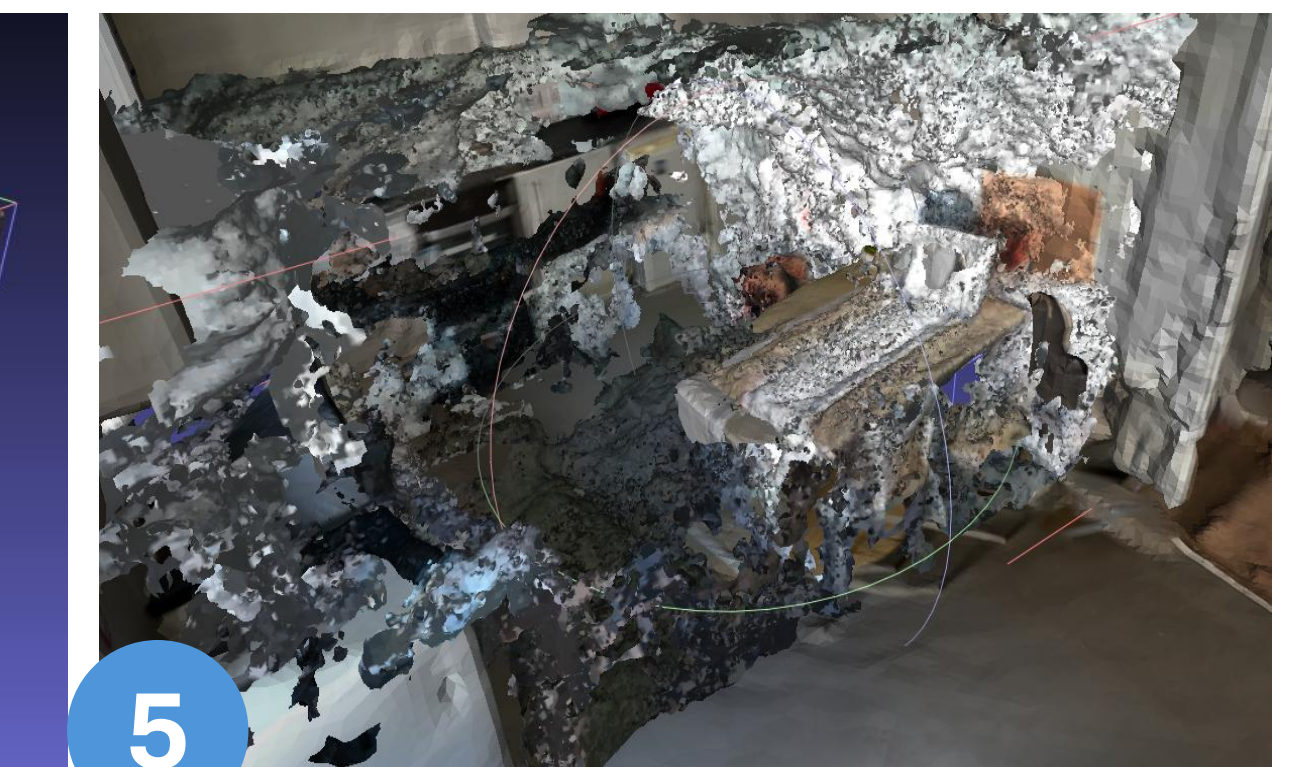
5 Register the mesh to the LiDAR scan to convert camera poses to metric scale
